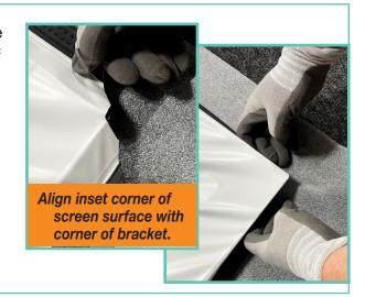
Attach the screen surface to the opposite diagonal corner of the subframe, and repeat on the other corners, as shown below.
