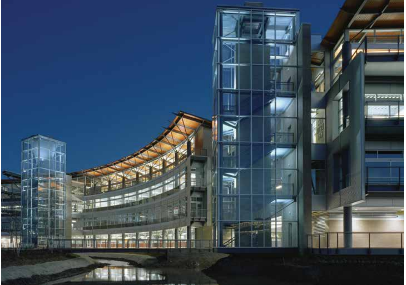
FlexShades®, Heifer International Headquarters, Little Rock, AR. Installation by Blind Ambition, Photography ©Timothy Hursley, Little Rock, AR., Little Rock, AR.
