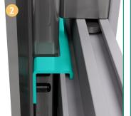
**Vertical rail hanger clips** allow installers to easily mount vertical rails.
